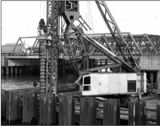
Fig. 11.26. Predrilling for a combined wall installation.
