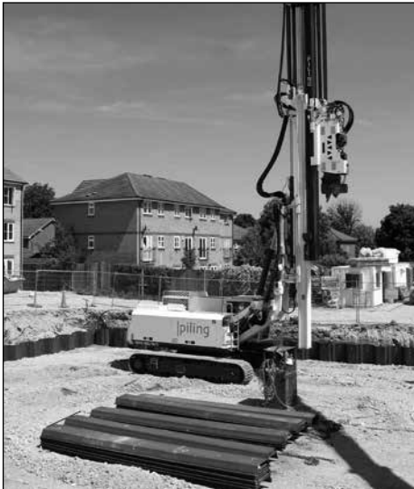
Fig. 11.13. Telescopic rig with vibratory hammer.
