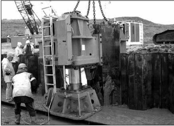
Fig. 11.18. Pile extractor.
