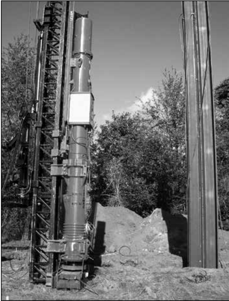
Fig. 11.6. Diesel hammer on fixed lead.
