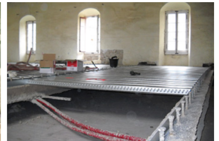
Installation within rehabilitation project - Cofraplus® 60
