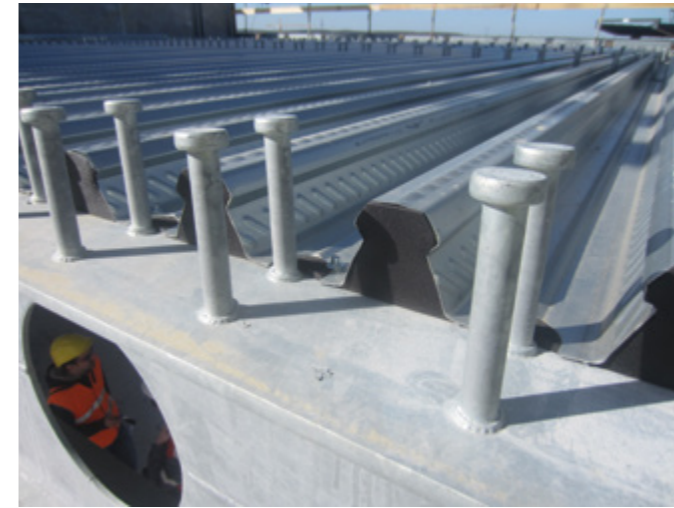
Cofrastra® 70 with profile filler installed on composite beam with double shear studs
