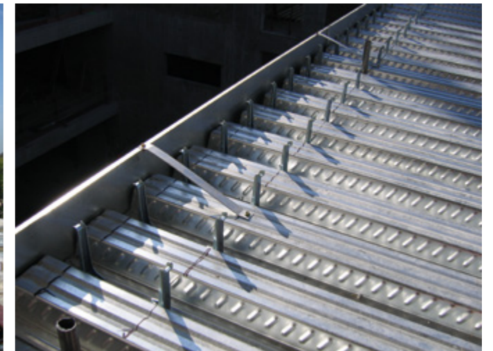
Edge trim with restraint strap and nailed shear studs
