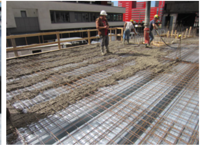
Concrete pouring on Cofraplus® 220 filling first the ribs
