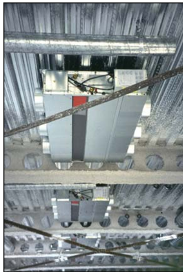
Figure 6.10 Cellular beams and service integration
