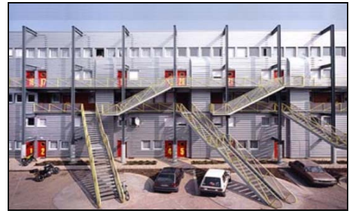
Steel cladding – Montargis (France)
