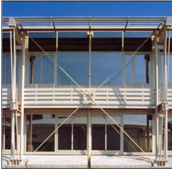
Figure 4.12 External cross-bracing in a multi-storey building
