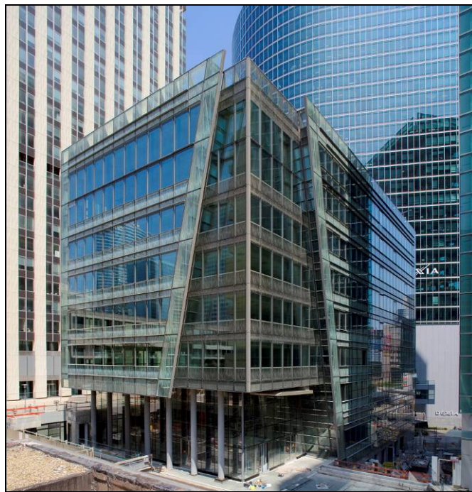
Figure 7.1 Praetorium building in La Défense (Paris) with 'High Environmental Quality' label
