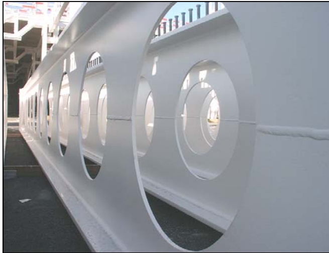
Figure 3.3 Cellular beams fabricated from hot rolled sections
