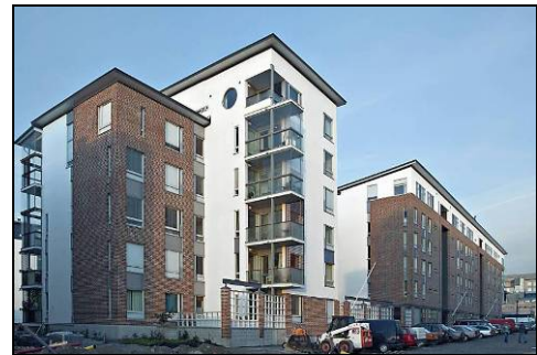
Render on load-bearing walls – Helsinki (Finland)
