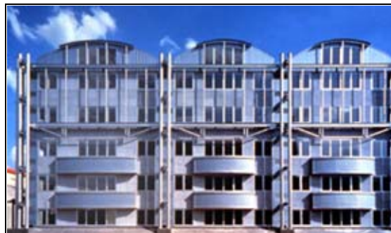
Figure 4.2 Building structure with tie members
