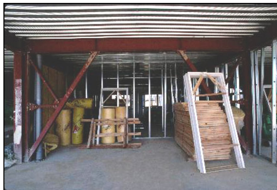
Figure 6.8 On site supplies with installation of plasterboards – Partitions and ceilings
