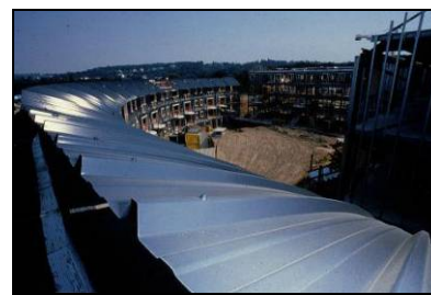
Pitched roof on site
