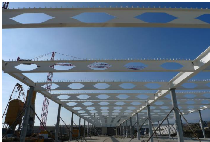
Figure 4.6 New type of beam – Angelina™ (composite beam), during erection
