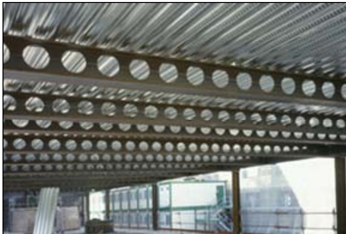
Figure 4.5 Composite cellular beams with steel decking
