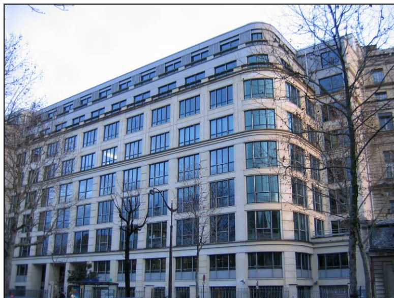
Figure 1.2 Office building in Paris
