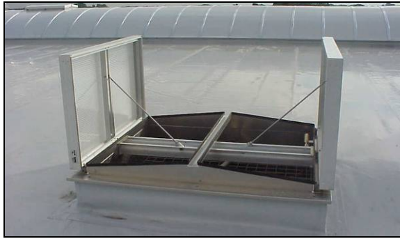
Figure 6.5 Smoke extractor
