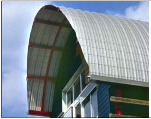
Figure 5.15 Curved roof with galvanized steel sheet
