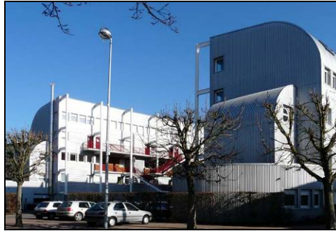
Steel cladding – Montargis (France)
