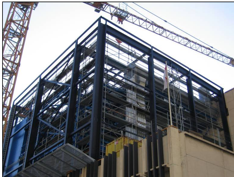
Figure 2.3 Multi-storey industrial building during construction, in Monaco
